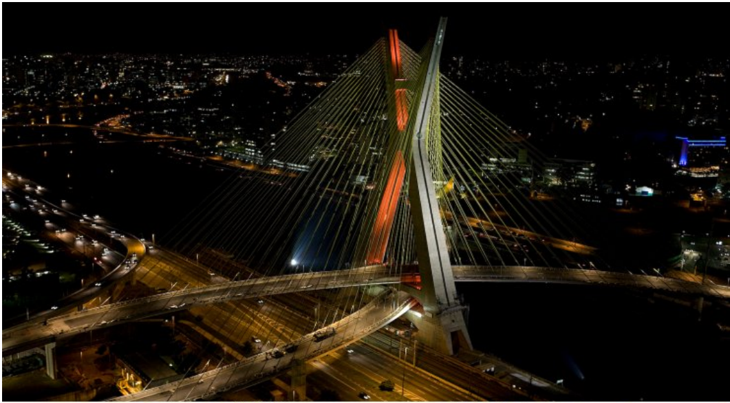
Octavio Frias de Oliveira Bridge, Sao Paulo, Brazil
